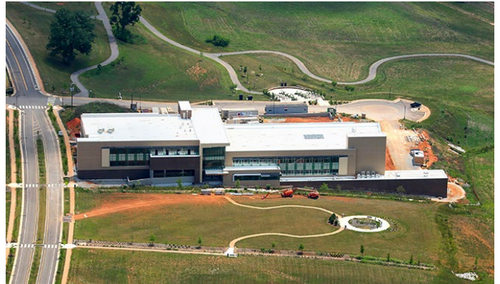
An aerial view of the Cherokee Farm Innovation Campus at the University of Tennessee. The first building at the site, the 142,000-square-foot Joint Institute for Advanced Materials, is nearing completion and should be ready for use by the end of the year, said Cliff Hawks, who is CEO of Cherokee Farm Development Corp.
